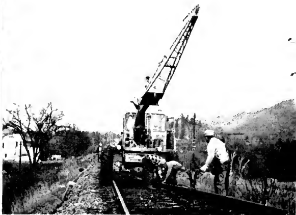
LAYING STANDARD RAIL
